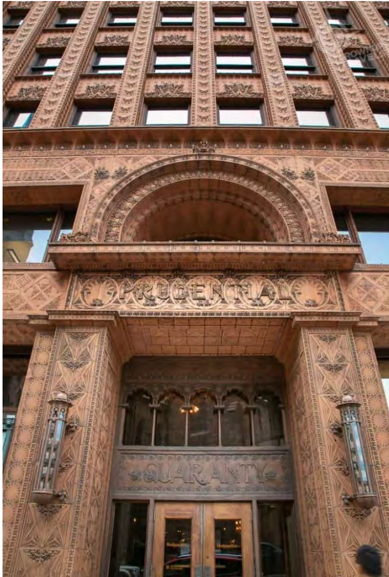
The Guaranty Building's main entrance, showing some of the details in the exterior terra cotta.
