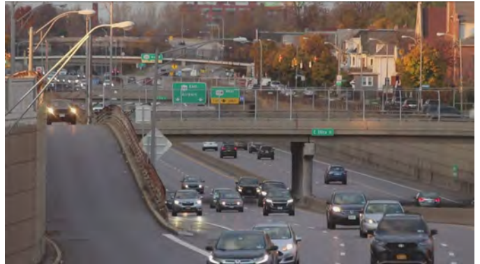
The Kensington Expressway, near Utica Street, 2024. (wgrz.com)
