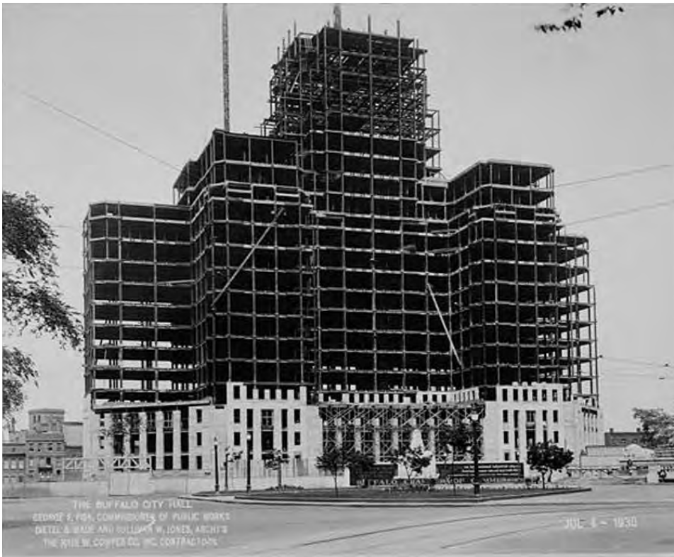
Buffalo City Hall under construction in 1930 (photo from buffaloah.com)
